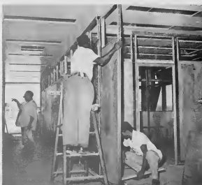
PUTTING up flexible birch partitions to form office walls was fairly simple. PONEMENTO di partiционnan flexible di berk pa forma muraya tabata facil.
